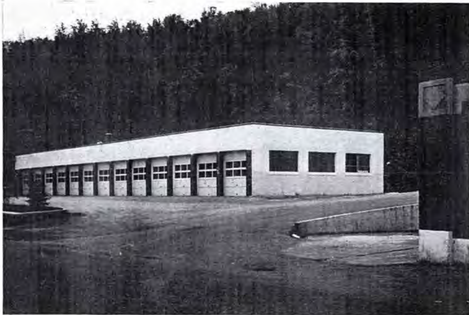
THE NEW GARAGE
